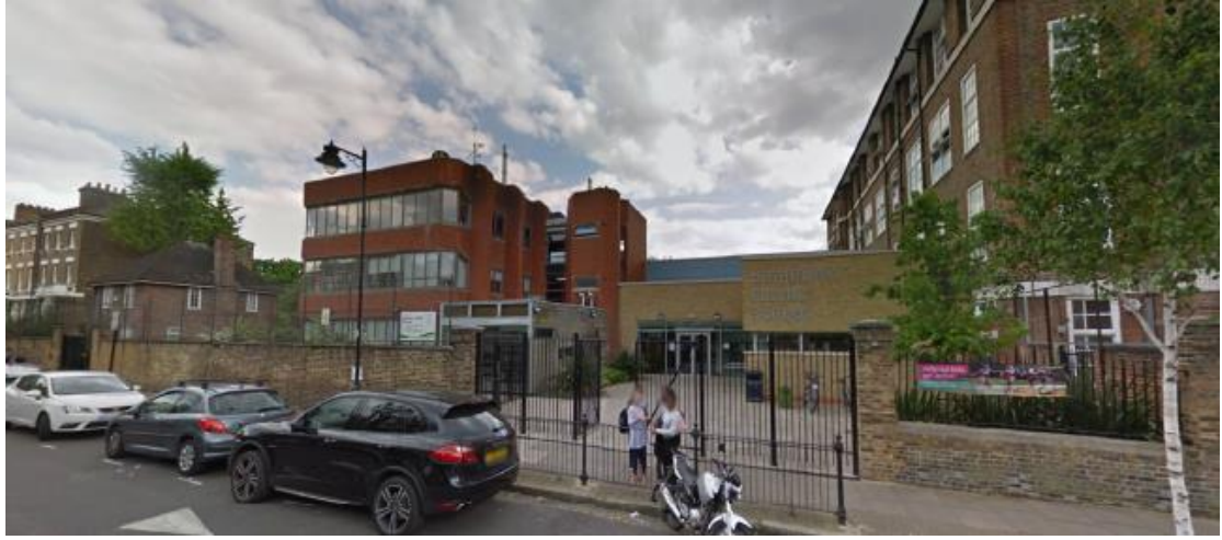
Image 3: View of the main school entrance
