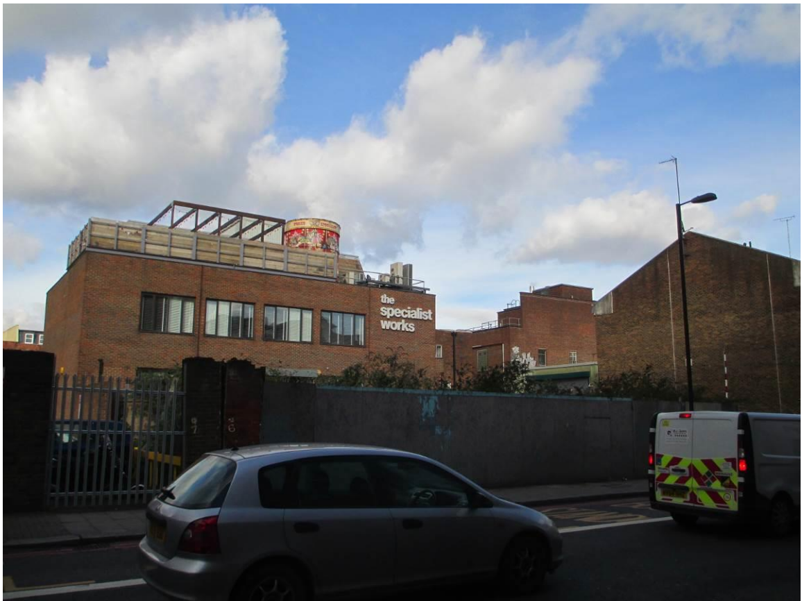
Image 3: Application site frontage
